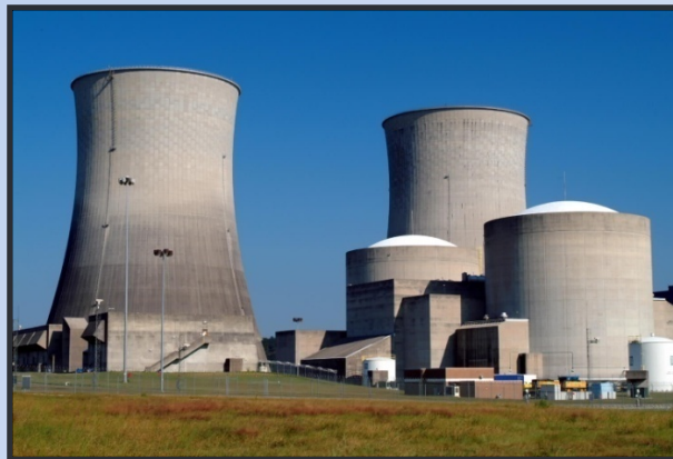
Watts Bar Nuclear Plant
