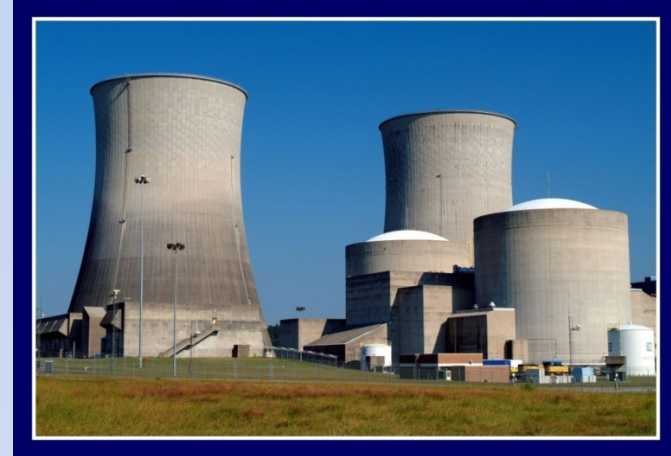
Watts Bar Nuclear Plant
