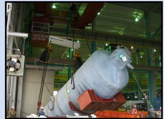
Moisture Separator Reheaters being lifted in the Turbine Building
