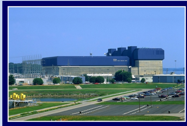
Browns Ferry Nuclear Plant
